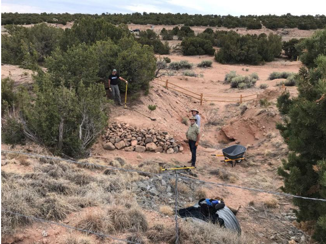
2020 grant recipient Santa Fe Conservation Trust. La Tierra Chili Line Trail - volunteers complete a retaining wall to support one side of a wooden footbridge (May 2021).
