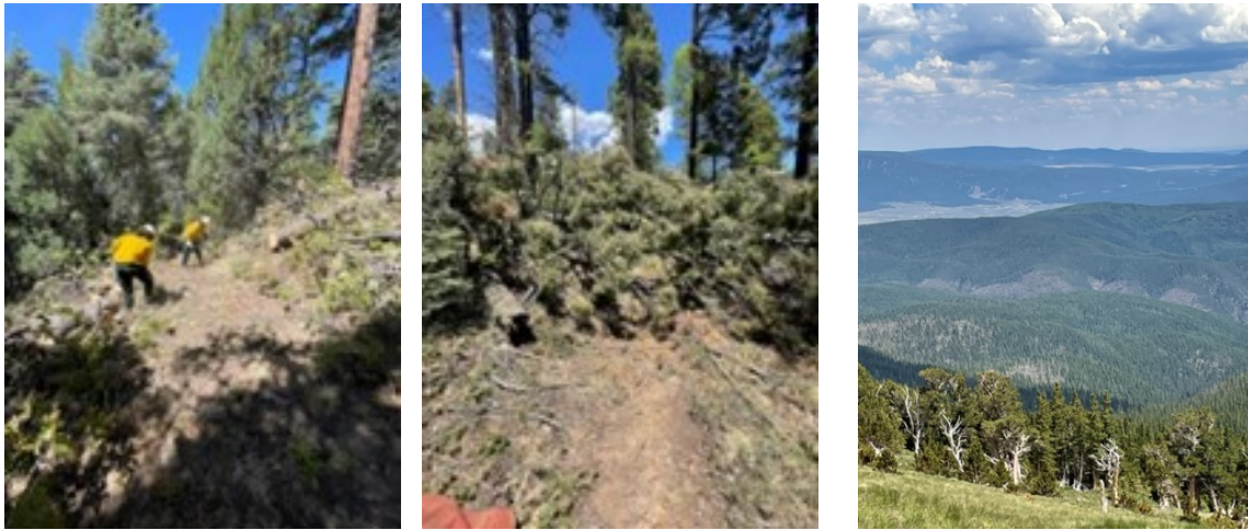
Taos Pueblo Trail Projects, courtesy of Taos Pueblo
