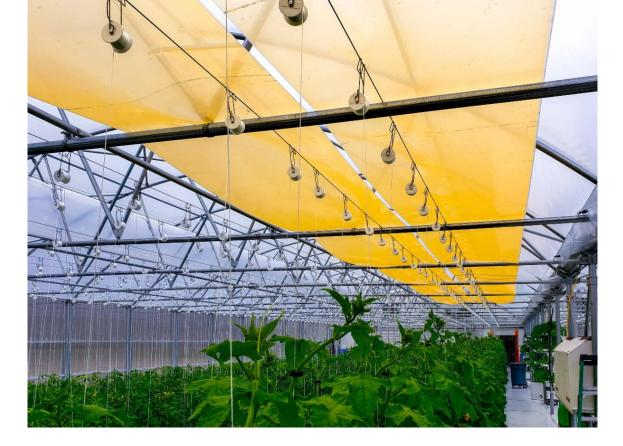
Installed above plants in a greenhouse, UbiGro®, UbiQD's first commercial product, is a layer of light that uses fluorescence to create a more optimal light spectrum for crops, converting under-utilized portions of sunlight to more photosynthetically efficient orange light that plants crave.
