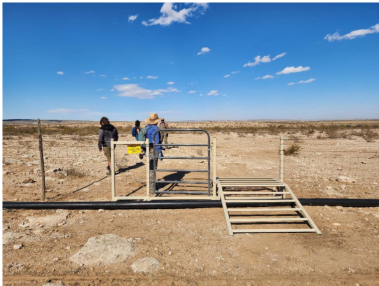
Cavern City Trail Keepers is installing 11 cattleguards and equestrian gates along the La Cueva Ridge Trail to connect the La Cueva Non-Motorized Trails System to the Guadalupe Ridge National Recreation Trail.
